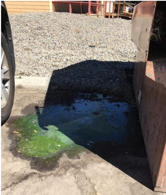
Photograph 4-3. Sewage Overflow in Public Parking Lot
