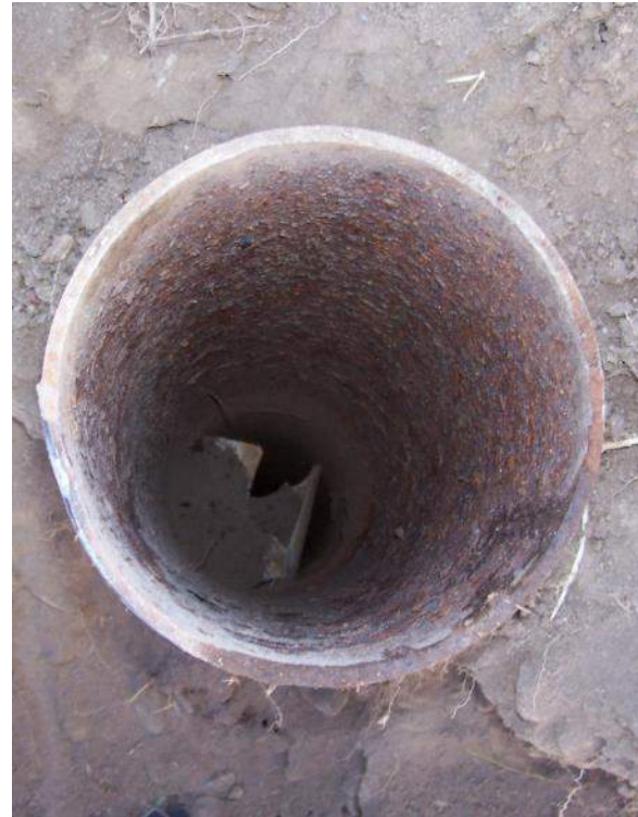
Photograph 4-4. Waste Disposal Well that Injects Sewage into the Ground
