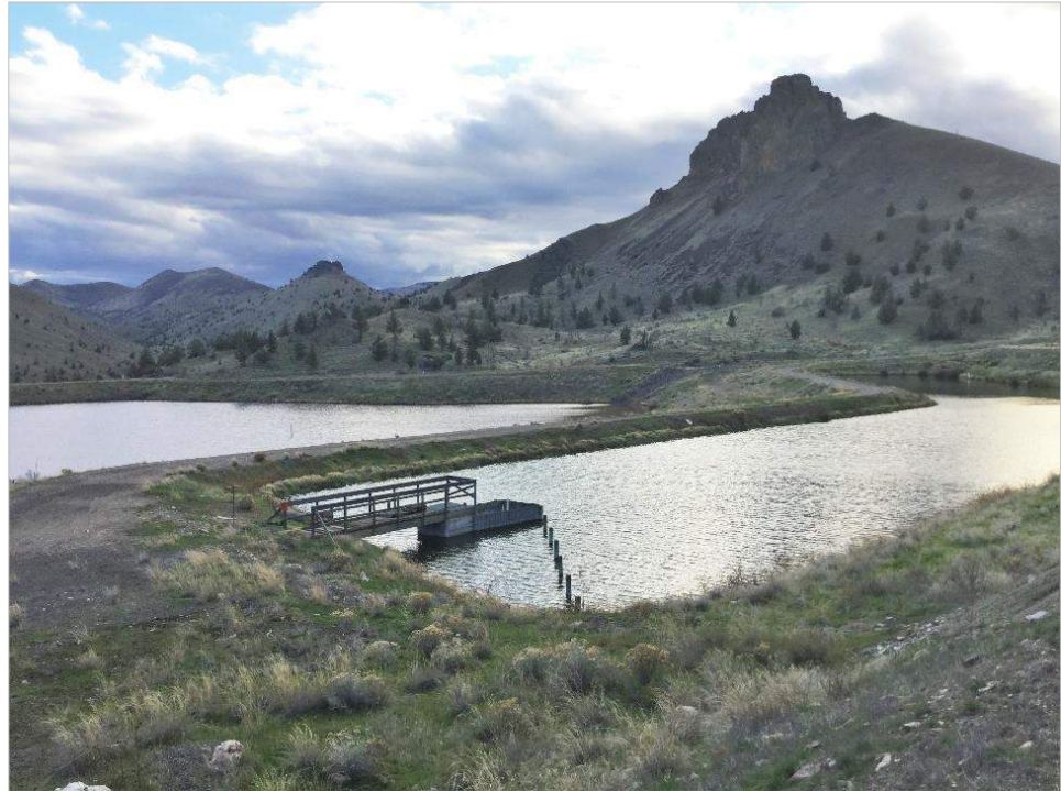
Photograph 5-1. Facultative Wastewater Lagoon in Eastern Oregon
