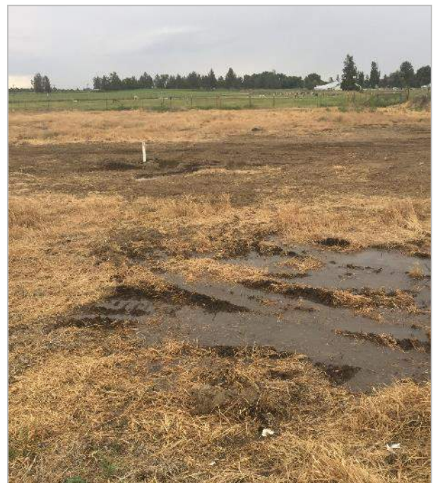
Photograph 4-2. Surfacing Effluent in Drainfield
